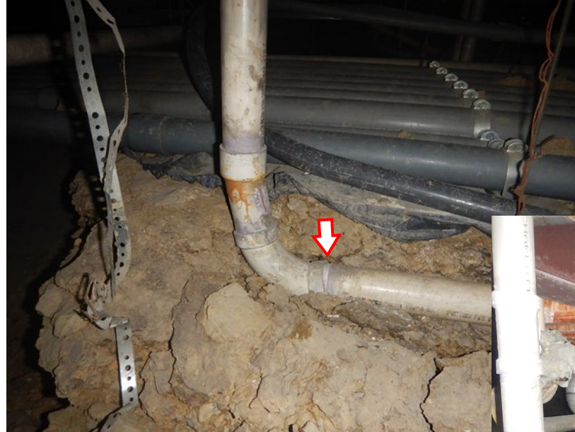
Cracked Plumbing
