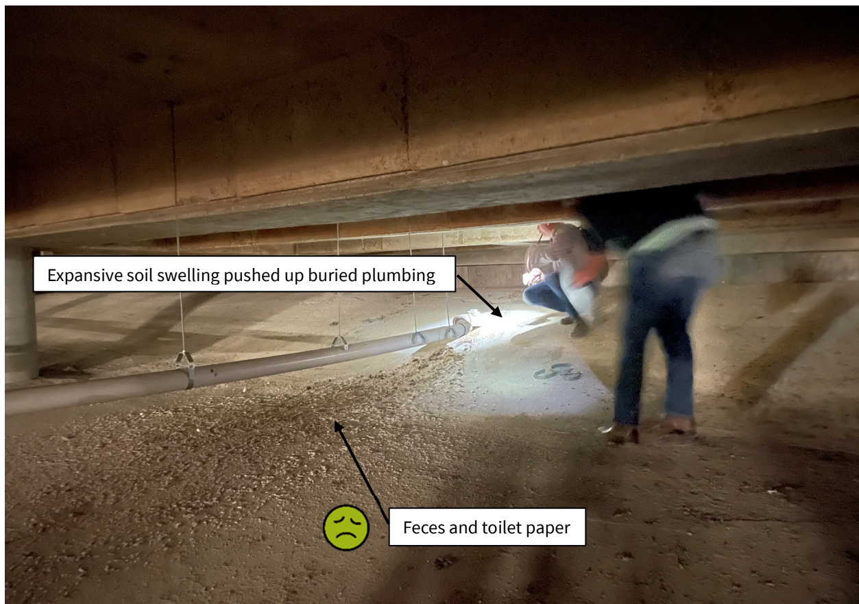
Photograph of a public school building in the San Antonio area of Texas, provided by a forensic engineer.
