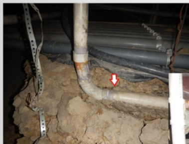
Cracked Plumbing
