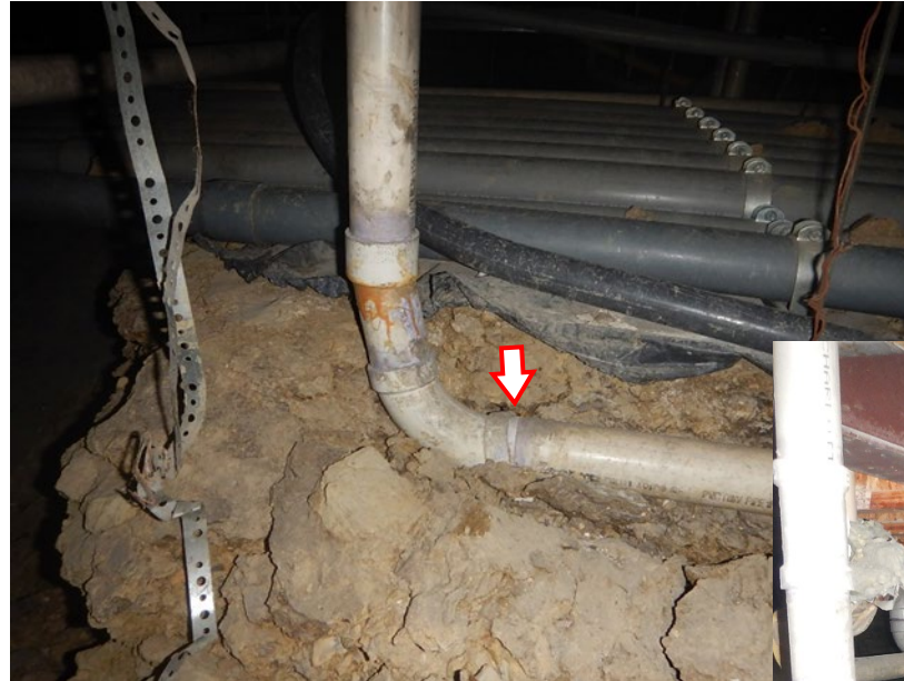
Cracked Plumbing
