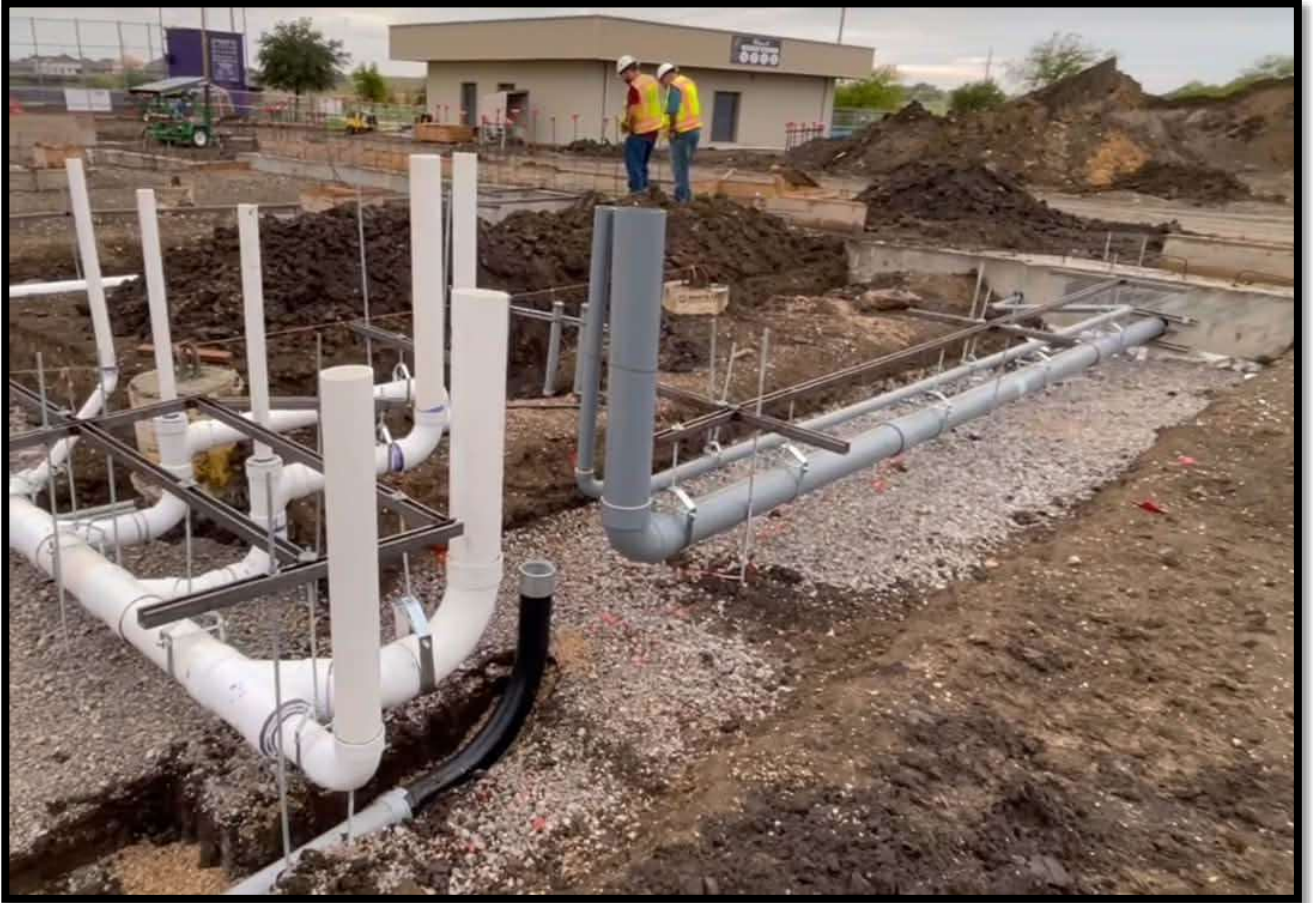
Figure 4.0-H Example of an in progress installation of Isolated Plumbing before Void Forms are installed. This image displays permanent framing members that will be embedded in slab and permanent plumbing with temporary vertical support rods that are to be removed after transferring support to rebar on carton forms, but before concrete is placed for the slab (pre-installed plumbing).
